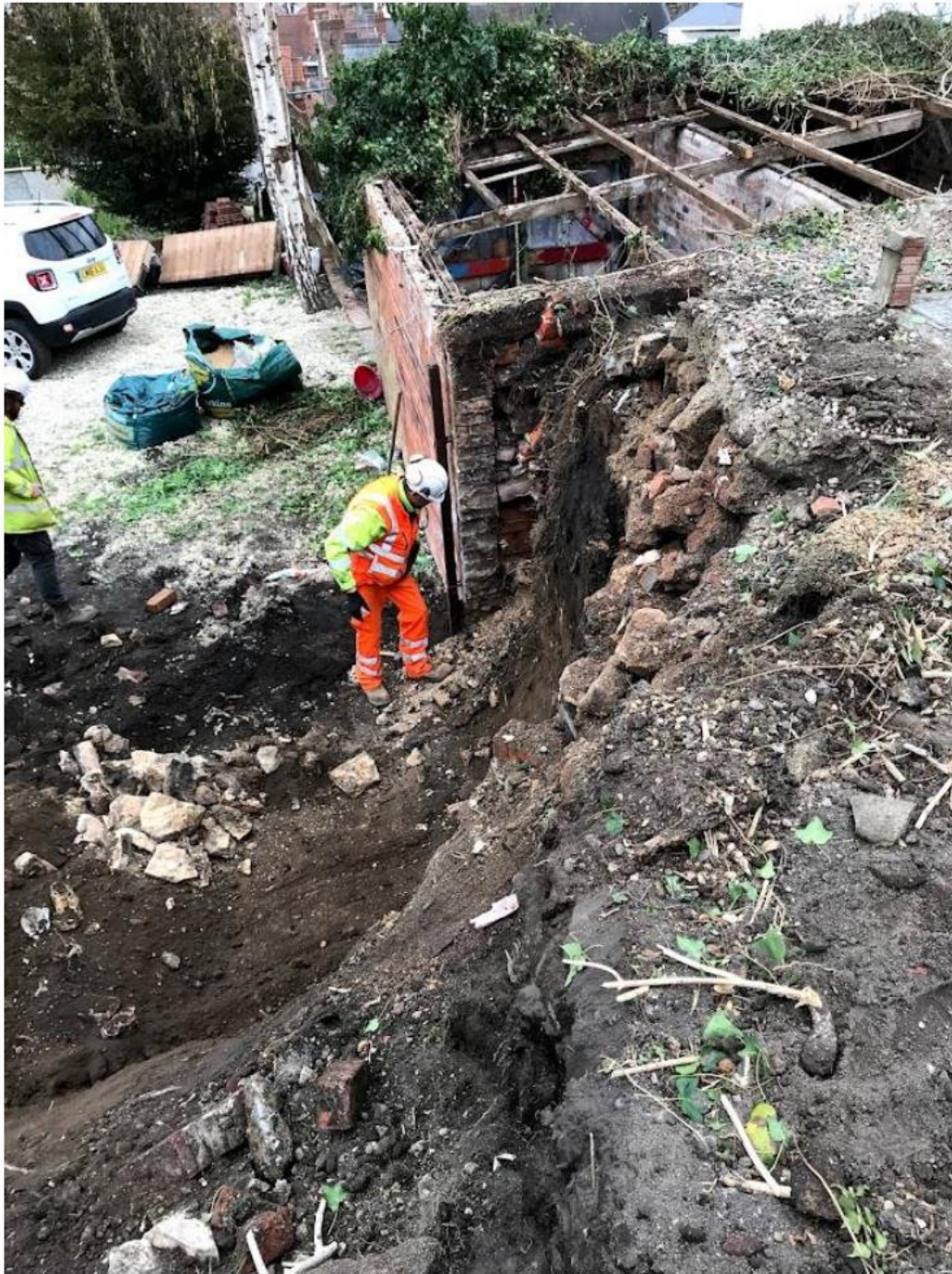
Clearly showing outbuildings are wall to wall abutting and therefore supportive to SAM retaining Northern wall.
