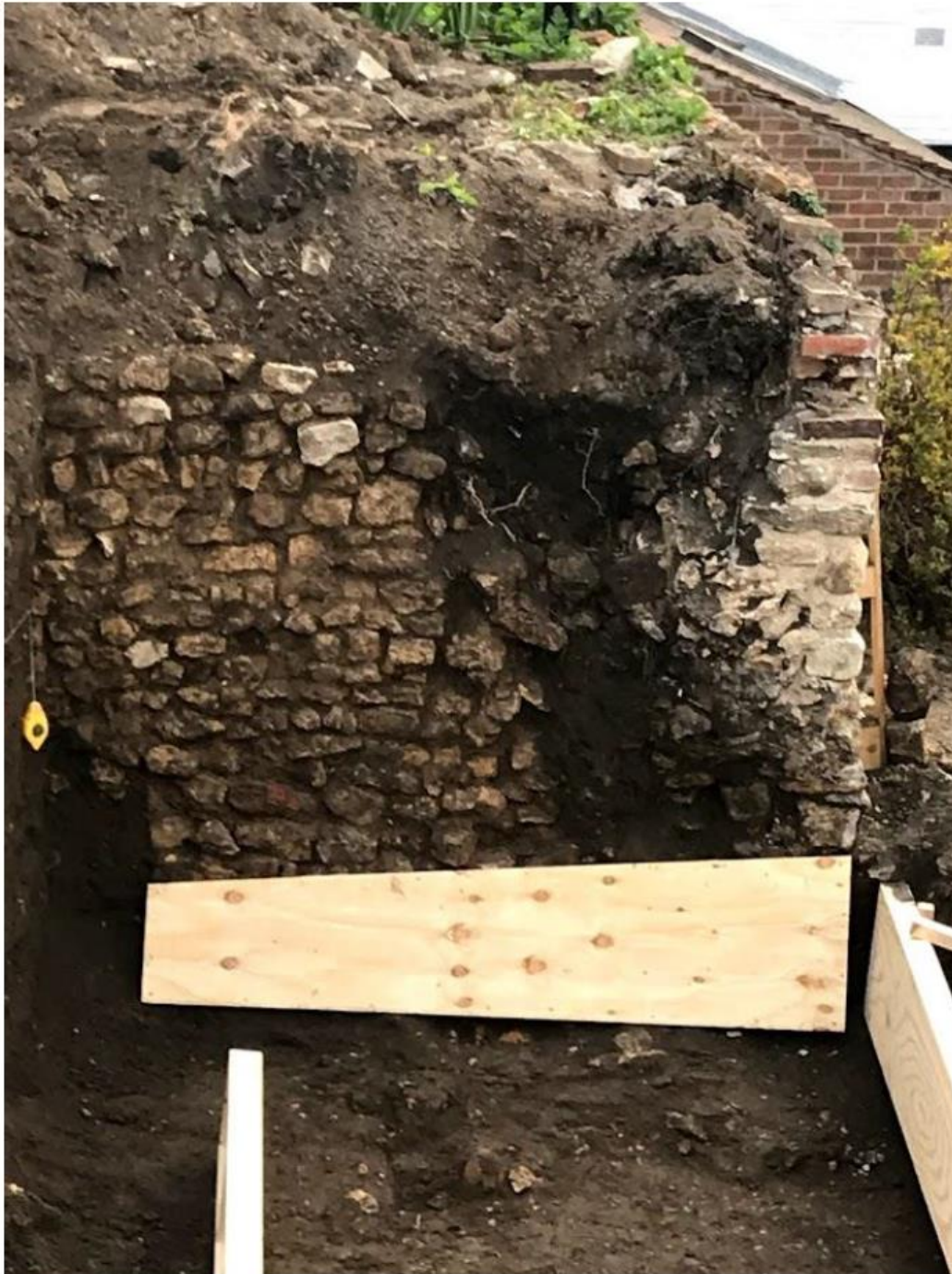
Northern retaining Stone wall cross section
